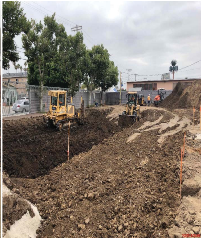
CO T-517 Removal of excessive soil moisture
