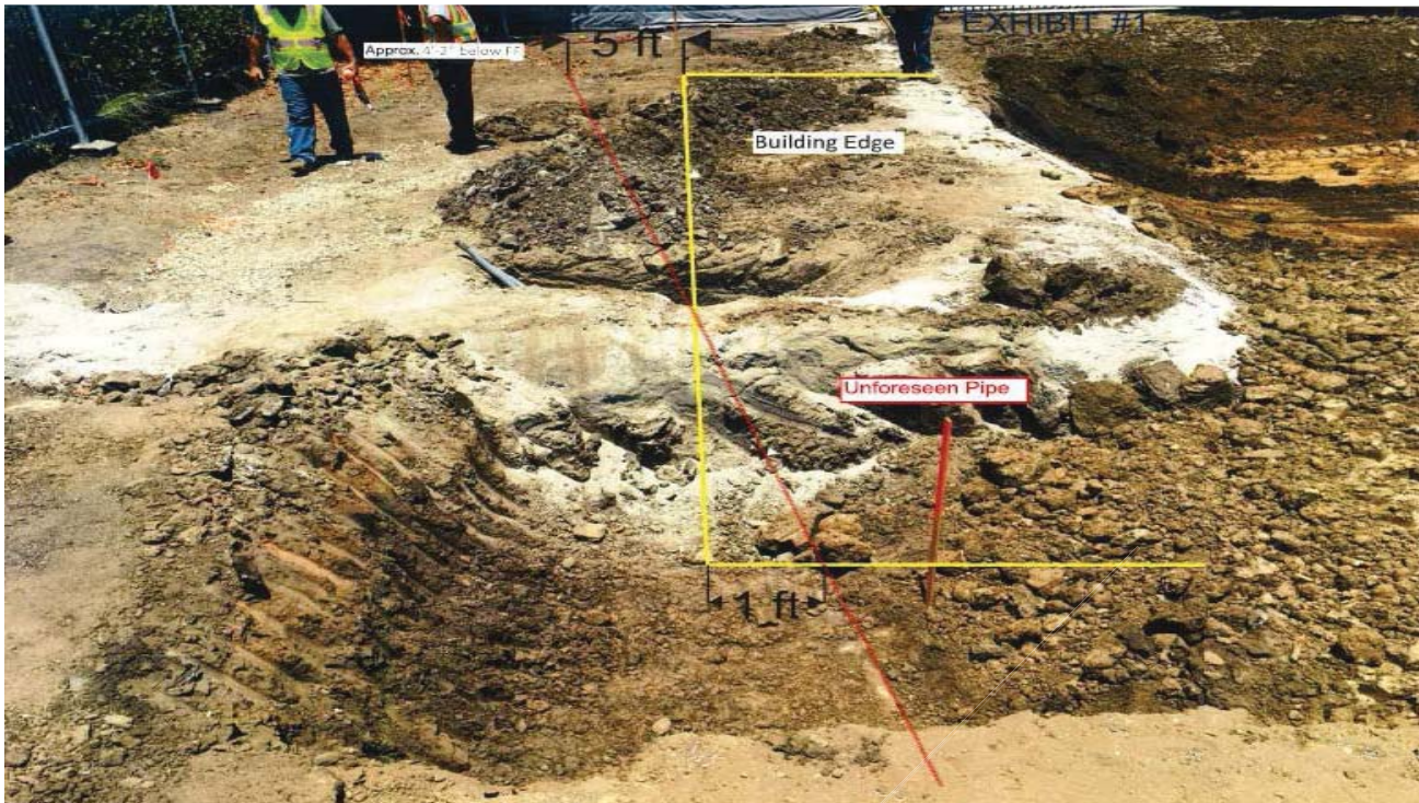
CO T-518 Removal of a segment of an abandoned pipe discovered during excavation
