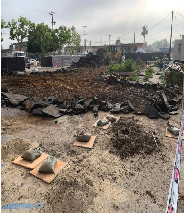
CO T-511 Demolition of asphalt concrete
